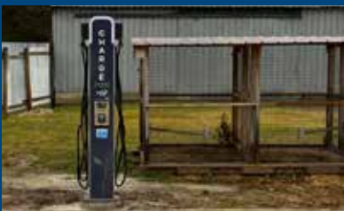
Level 2 EV Charger Installed at Osborne Nature Center in Elkader
